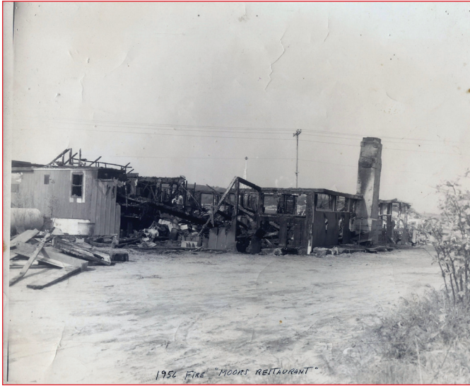
The Moors Restaurant after the fire, May 28, 1956
