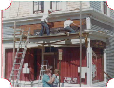
Dick and Robert Henrique renovating Vorelli’s Restaurant, former Matta’s 5¢ & 10¢ Store.
