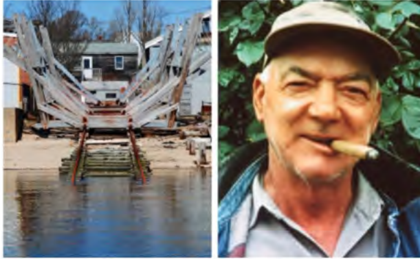
Left: Head-on view of the marine railway at Taves Boatyard shows the tracks running out to the harbor and the cradle in which boats are hauled to dry land. Right: Frank “Bisca” Taves in an undated photograph from Bill Berardi’s “Faces of Provincetown” collection, assembled and scanned at Provincetown High School, under the direction of Judith Stayton, and held by the family of Gordon Ferreira.
